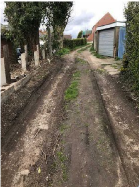
Fig. 17 Unstable condition of Victoria Passage surface where it is bare earth and deeply rutted.
