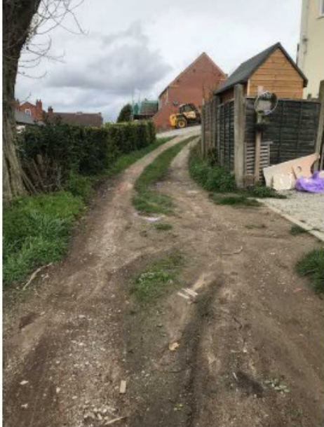
Fig. 16 Poor condition of Victoria Passage surface. Note the close proximity of Victoria Passage to the Alexandra Terrace property (on the right of the image). Note also how narrow and steep Victoria Passage is at this point.
